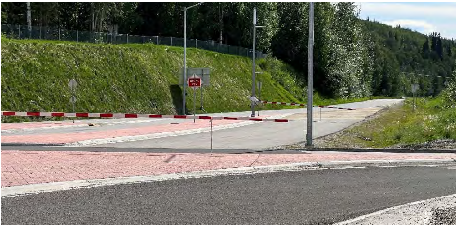
Looking South-East Ramps (Northbound Off-Ramp) By-Pass Lane and Gates
