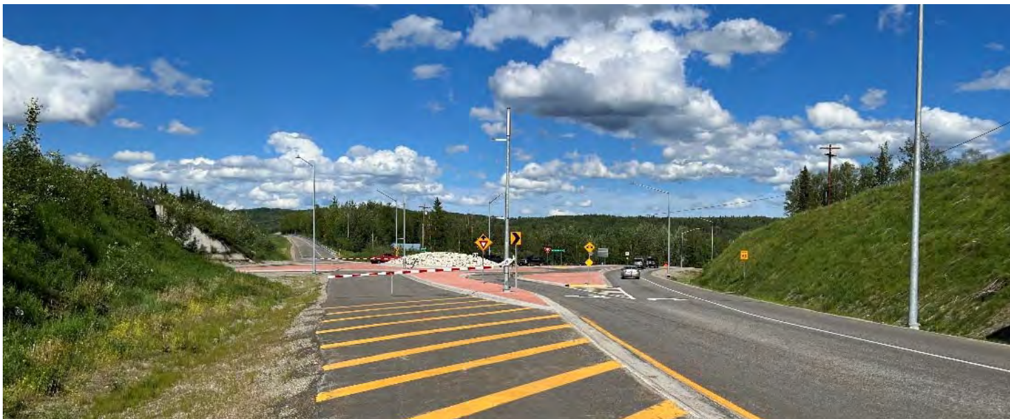
Looking North-East Ramps (Northbound Off-Ramp, nearside; and On-Ramp, far side) By-Pass Lane and Gates
